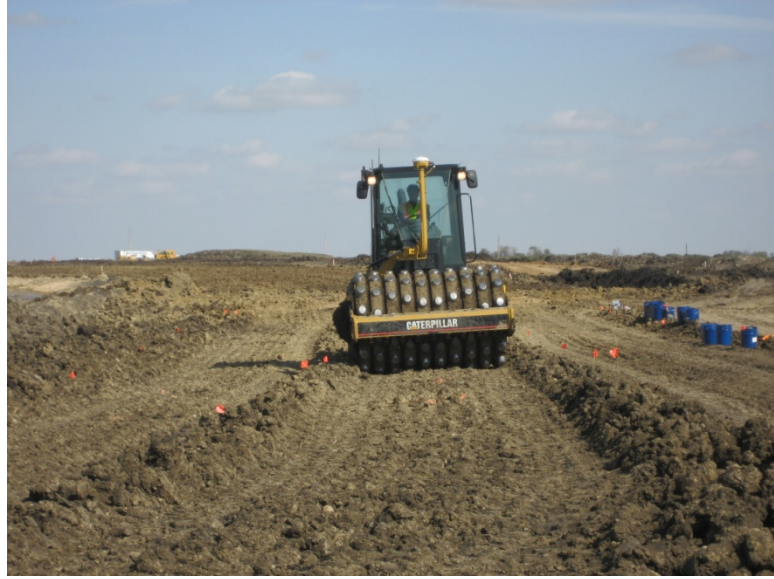
Figure 76: TH60 strip compaction
