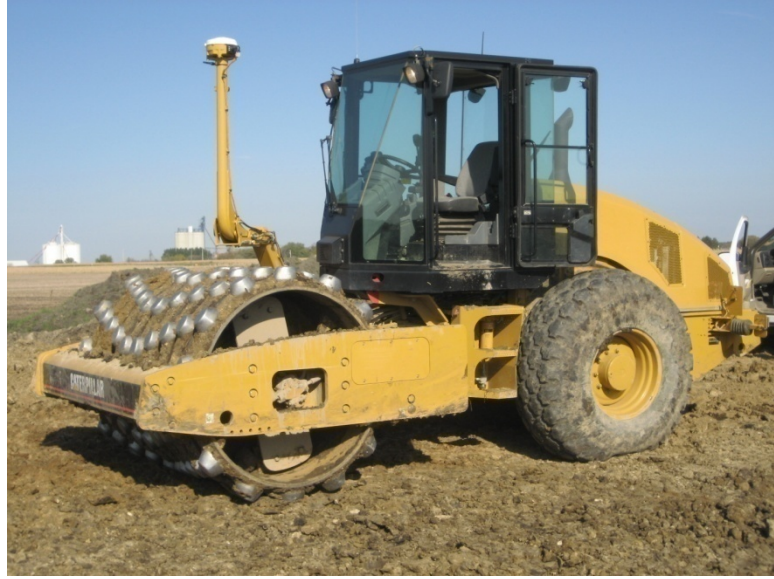
Figure 26: Compactor used for TH60 project (specifications unknown)
