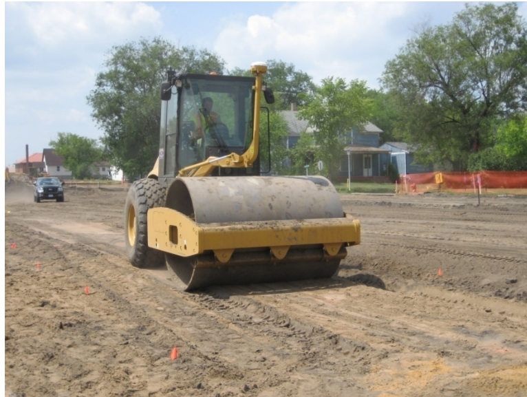
Figure 75: Field compaction using CS-563 roller
