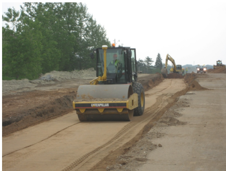
Figure 74: Field compaction using CS-563 roller
