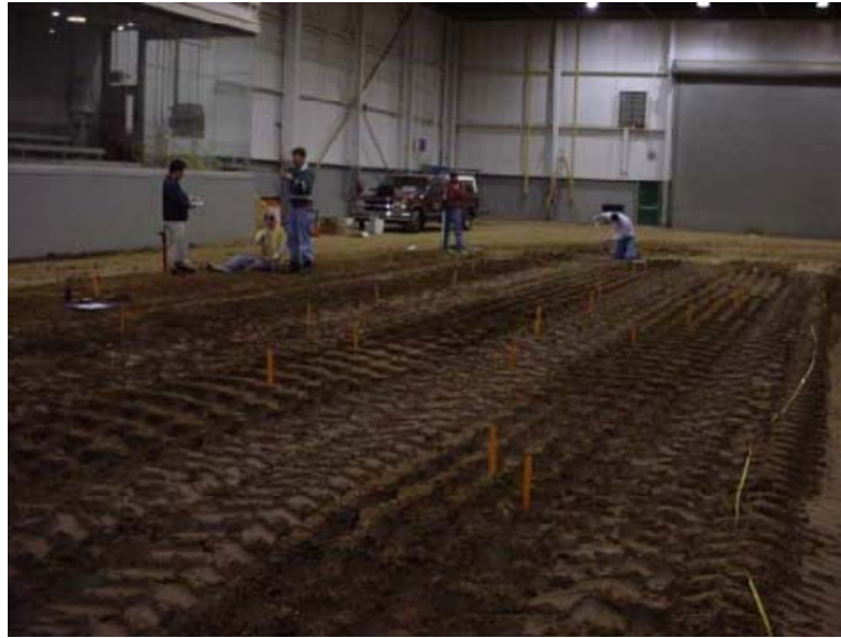
Figure 69: Test strips A through D after compaction
